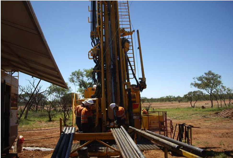
Figure 2: DDH1 Drilling with Sandvik 1200 Multipurpose AWD truck mounted rig set up on hole EL15D01 at Artemis.
